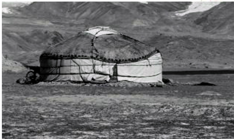
Mongolian YURT with collapsible “pantograph” side walls, and felt mat covering.
